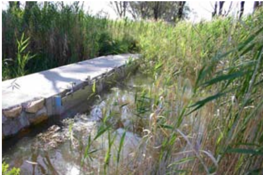
Figure 2. Photograph of regulator on the downstream inlet in Martin Bend.
