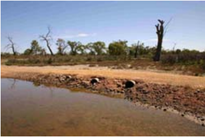
a) Three pipes under track at Causeway 1
