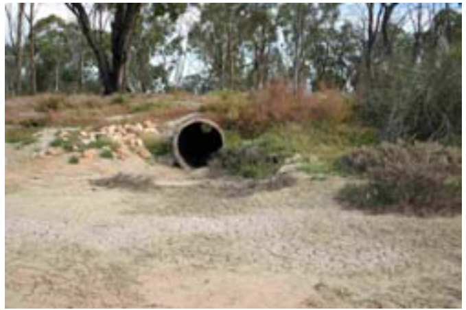
b) Pipe between permanent and temporary lagoon
