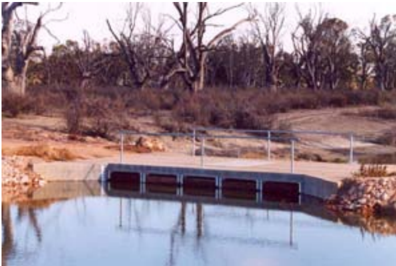
Figure 3. Photograph of the Overland Corner regulating structure (2004).
