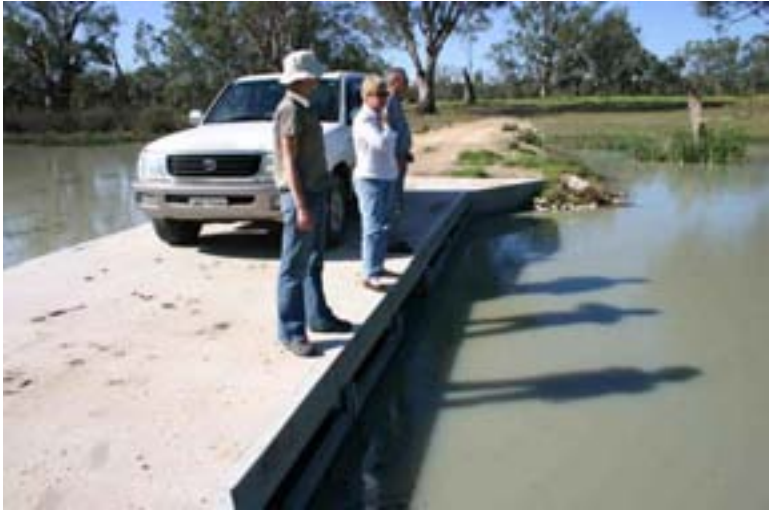
Figure 3. Photograph of the Beldora Wetlands regulating structure.
